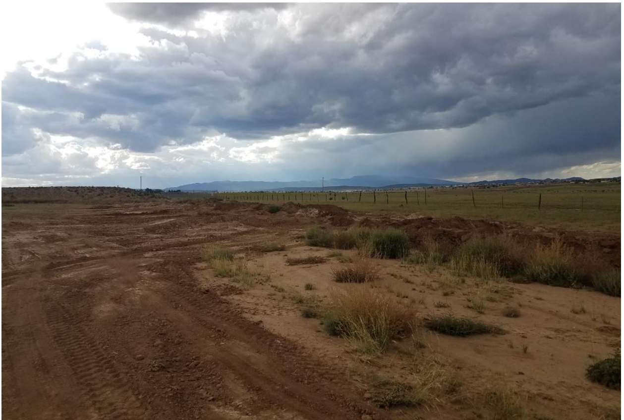
c) See the attached photo showing that the additional ponding areas have been dewatered and are in the process of being backfilled and regraded.
